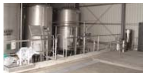
In acht Bodentanks mit jeweils 20.000 Liter Fassungsvermögen lagern explosive Stoffe. Explosive substances are stored in eight floor tanks each with a capacity of 20,000 litres.
