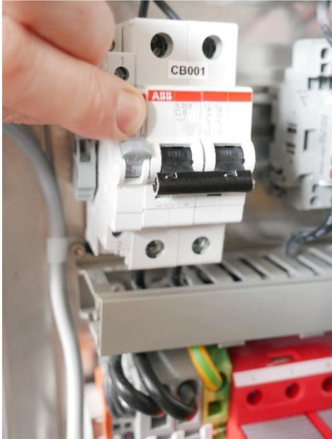
Figure 11: Switch position up for UPS on
