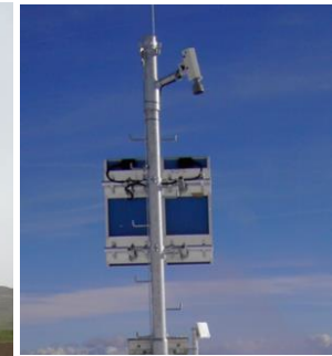
Solar powered SHM30 snow depth station.
